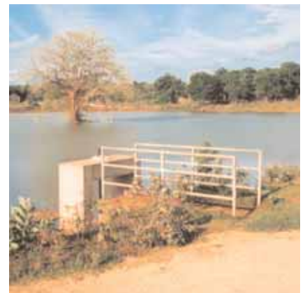
One of the new small tanks at Uda Walawe Left Bank
