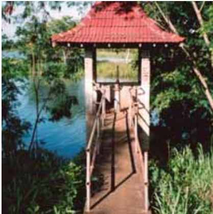
Sluice of reinstated tank Uda Walawe
